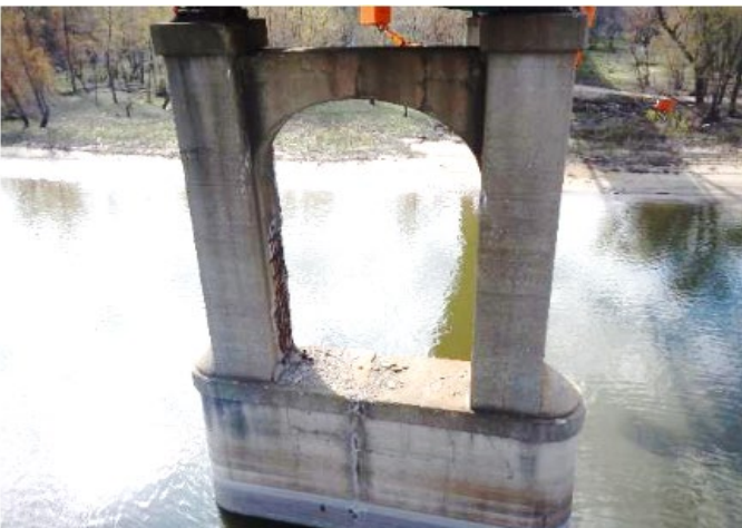
Photos from the latest bridge inspection illustrating deterioration and corrosion.
