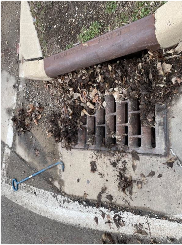
STA 48+85 (RT): Inlet at SE Quad of 3 rd St (IL 18) and School St
