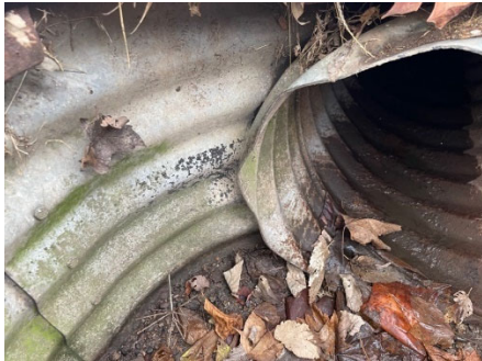
STA 55+05 (RT): EX Yard Inlet w/ CMP connections and build.
