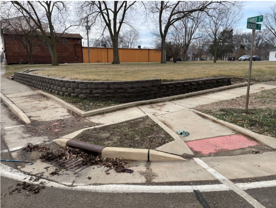
STA 48+08 (RT): Inlet at NW Quad of 3 rd St (IL 18) and School St
