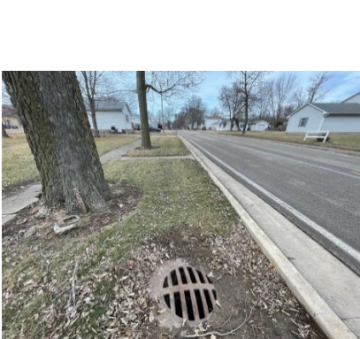
STA 52+85 (RT): EX Yard Inlet note CMP connections and build.
