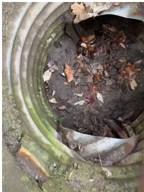
STA 52+85 (RT): EX Yard Inlet note CMP connections and build.
