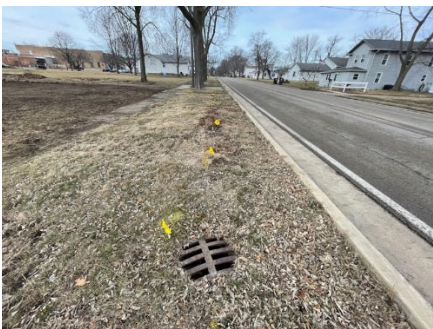
STA 55+05 (RT): EX Yard Inlet w/ CMP connections and build.
