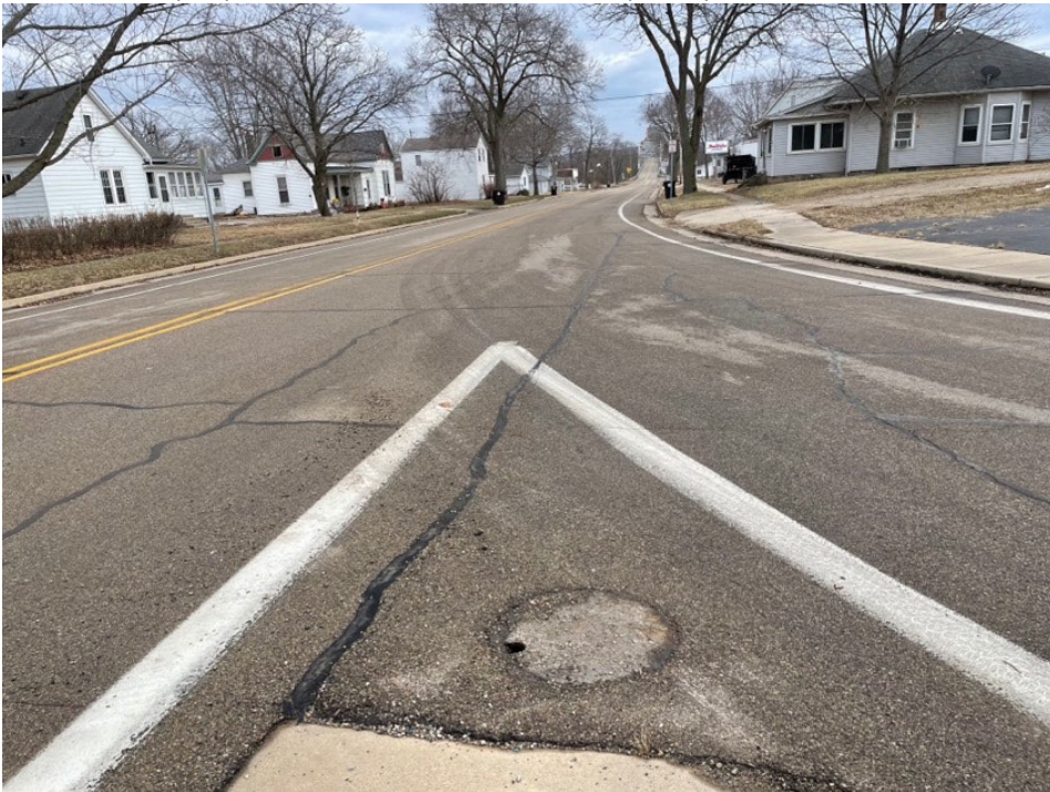
STA 48+82 (RT): Traffic Island & SS MH at SE Quad of 3 rd St (IL 18) and School St
