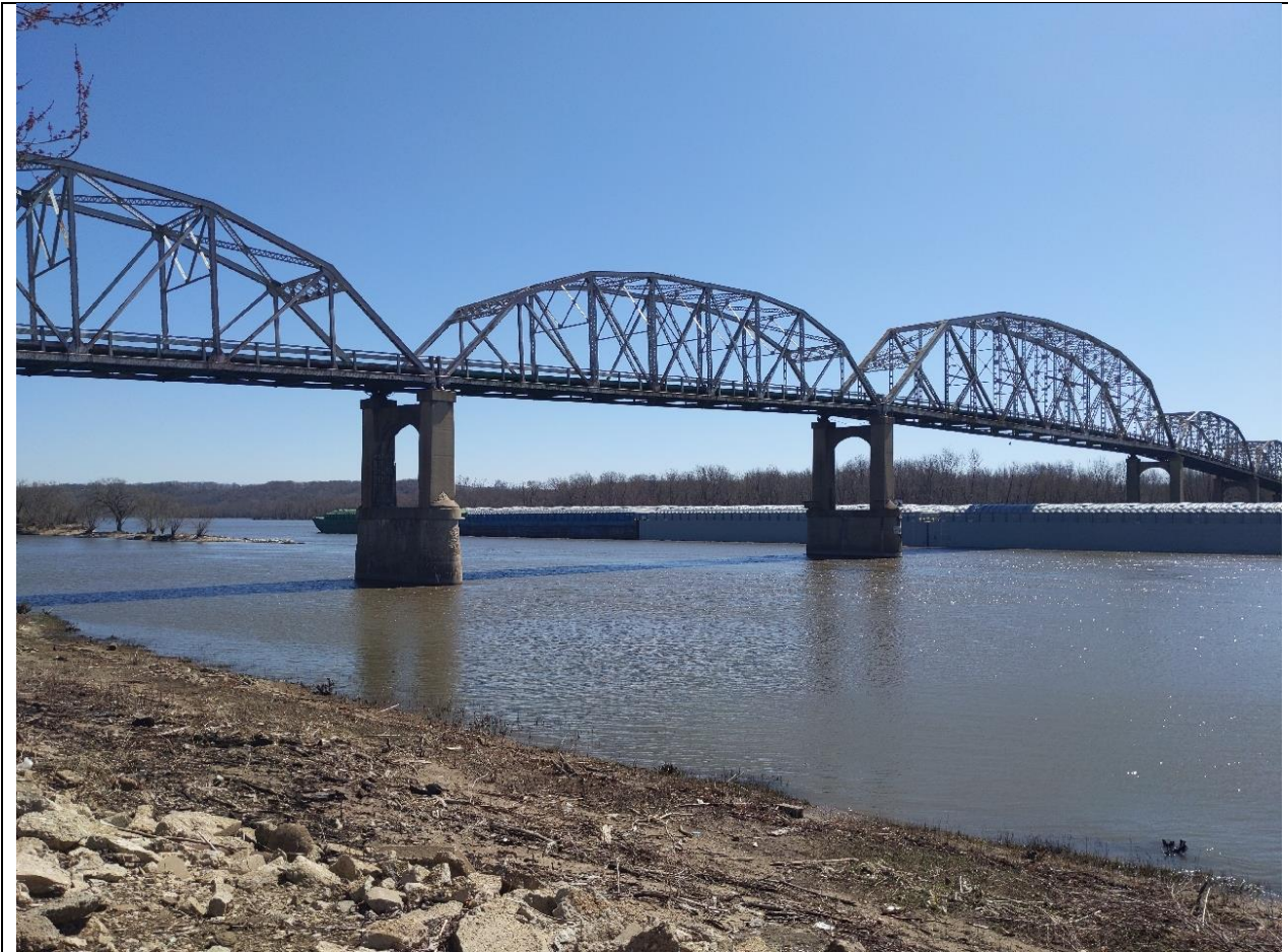
Photo 5 - Looking east. A tow of covered hopper barges being pushed upstream through truss span 5.
