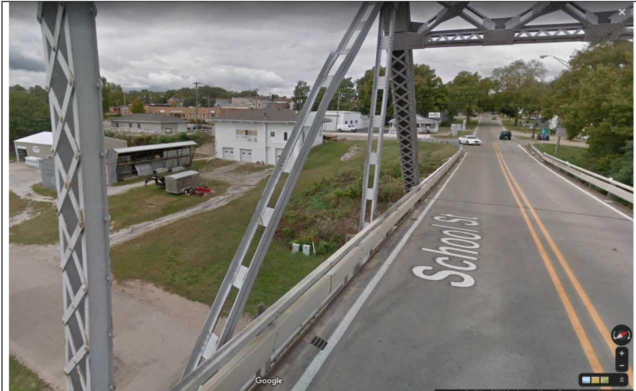
Photo 8 - Looking north. Entering Henry from the bridge.
