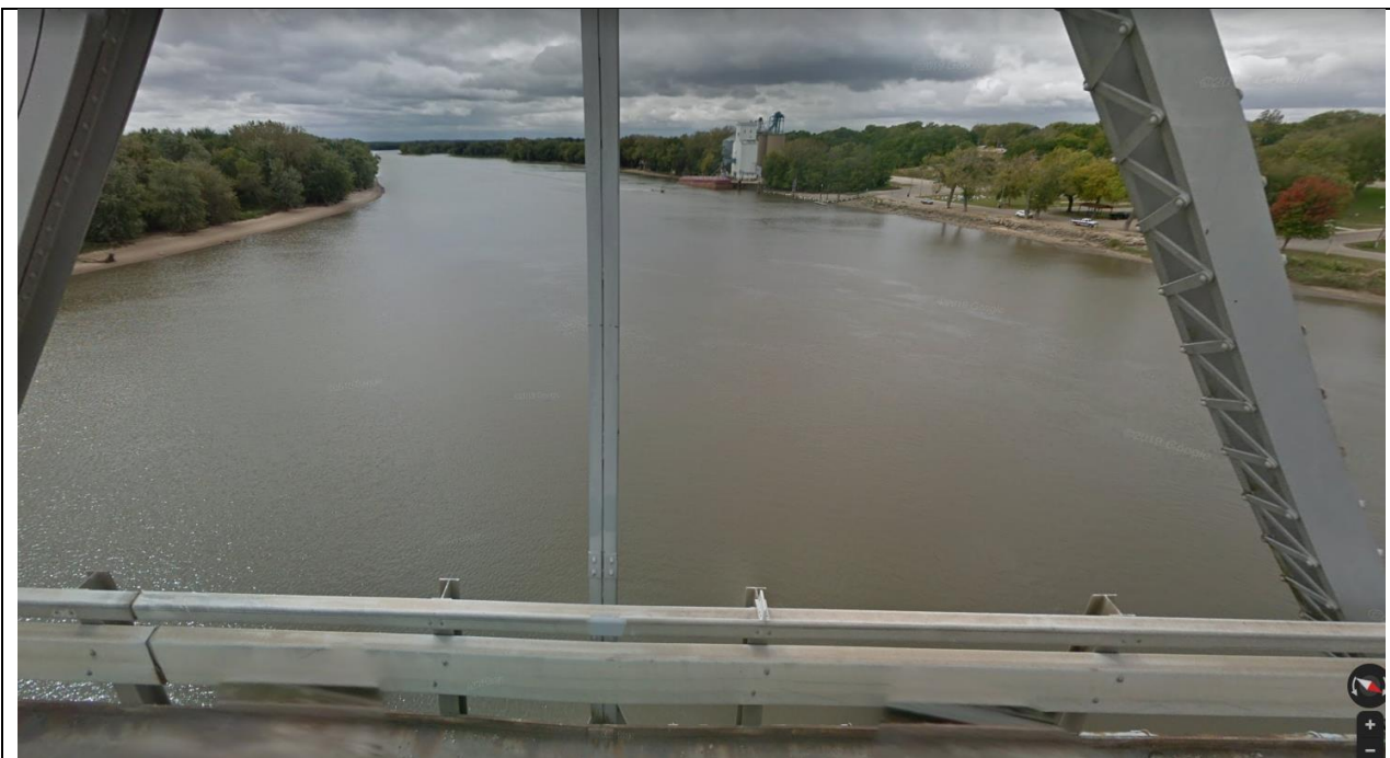
Photo 7 - Looking west (downstream). Henry waterfront and grain elevator at right.
