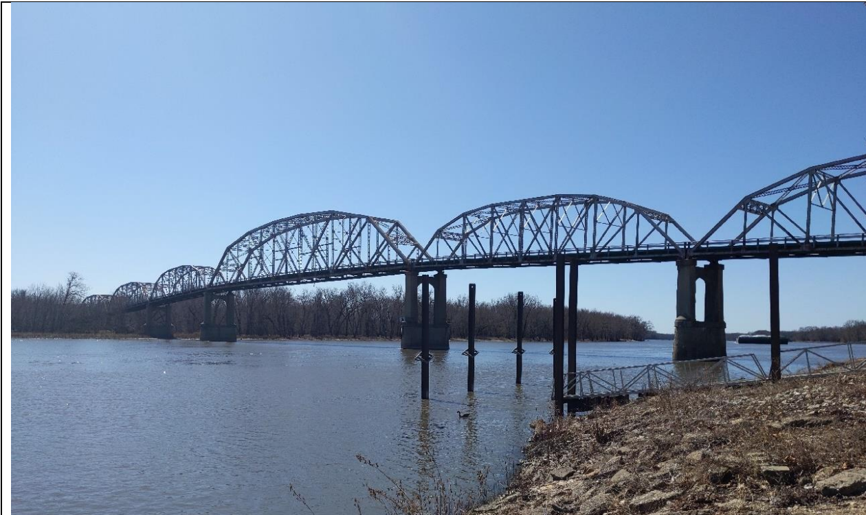
Photo 3 - Looking west. Spans 3 (partial at right), 4, 5 (navigation), and 6 leading into the trees on the south bank at left.
