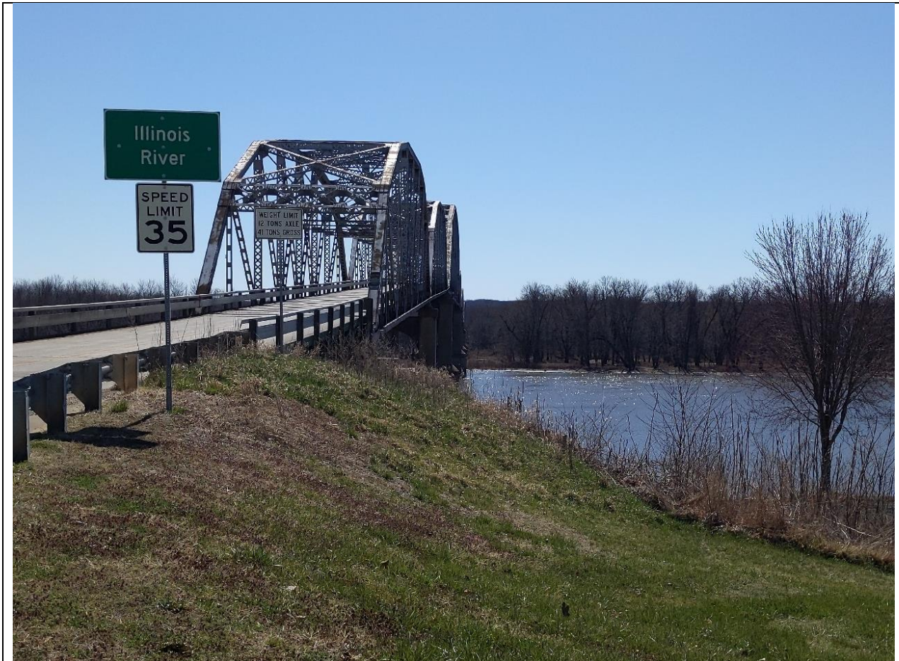
Photo 1 - Looking south from Henry. Approach spans 1 and 2 and truss span 3. Note posting sign restricting bridge to legal loads only.
