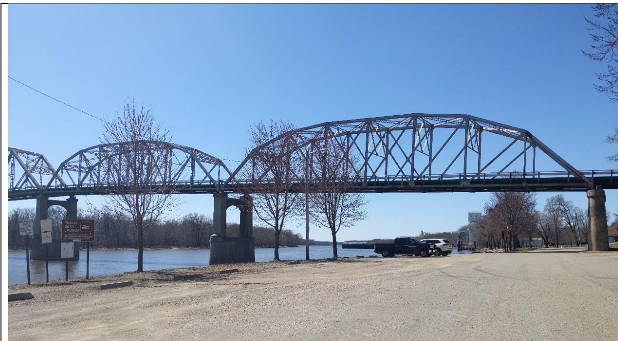
Photo 4 - Looking west. Truss spans 3 and 4. Cromwell Dr. passes under span 3 at right.
